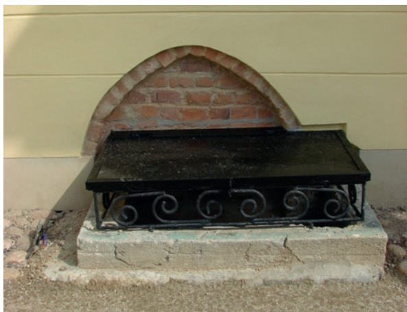
33. Pointed arch basement window in the garden elevation of the palace [W. Paszkowski, op. cit., p. 287].
